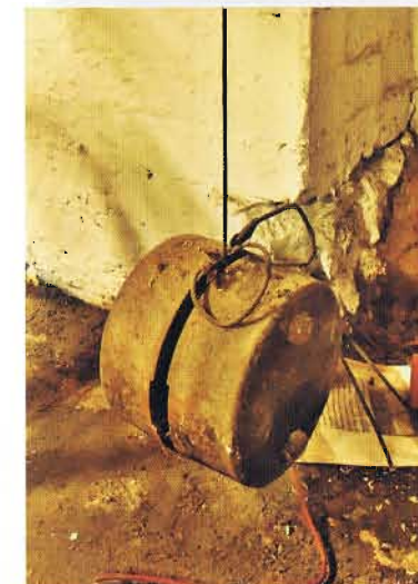
A weight still hangs on the house curtain guide wire after 55 years
